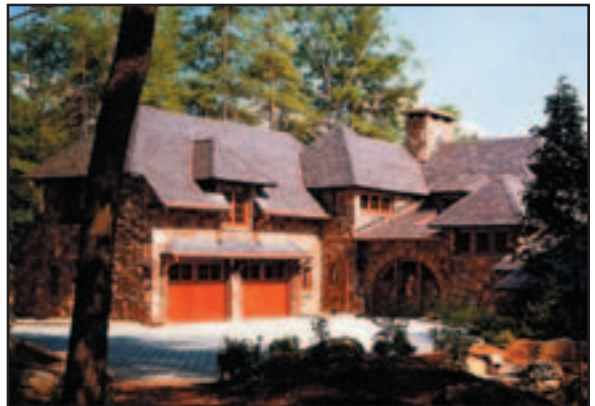
Sensitive thought must be given when locating the garage. The roof massing and detailing help downplay the potentially overwhelming presence of the garage. The front door remains the focus as one approaches the house.
