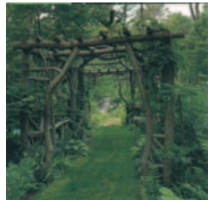
This arbor is constructed from Locust wood and has a rustic quality. This character, and the appropriate use of materials such as Locust, are encouraged.
