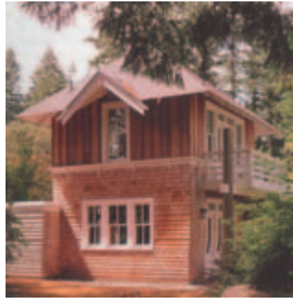
Guest cottages shall have the same architectural character as the house proper. The board and batten siding over the shake siding provides a nice textural contrast and reinforces "woodsy" character of the home.
