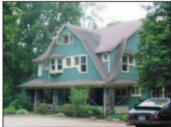
The roof massing and recessed porch are hallmarks of the Shingle Style. The bay windows and gambrel roof add to the character of the home.
